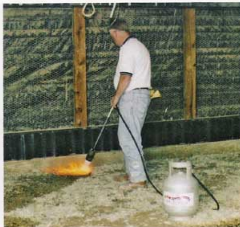
A hand-held torch is used to apply heat along the edges of the poultry shed's walls and corners. Photo courtesy of the Oklahoma Propane Gas Association.
